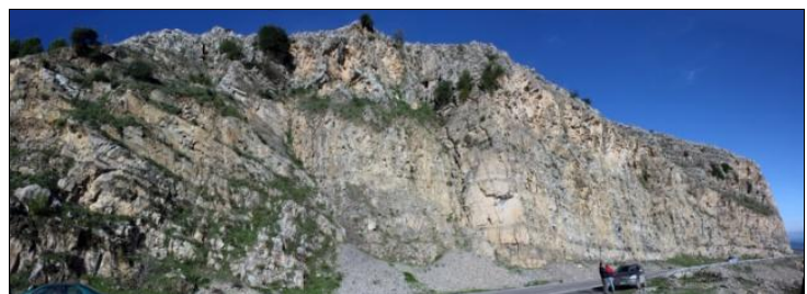
Figure 7. Zone de broyage RN 80 Pk 71+100
